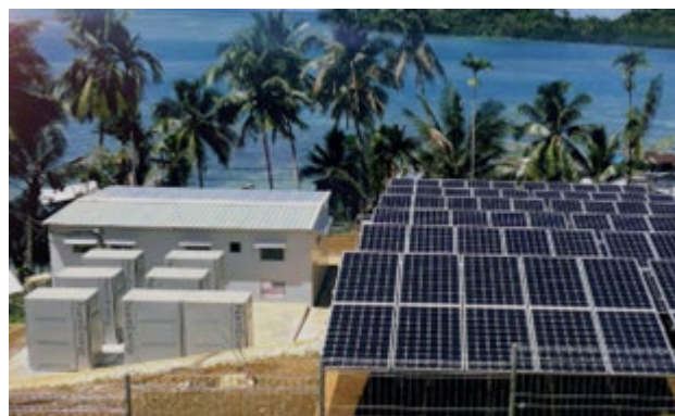
Fig. 7. a) Principle of operation of the rechargeable metal air battery. b) Nantenergy zinc-air-battery for solar energy storage (with permission of Nantenergy, USA).
