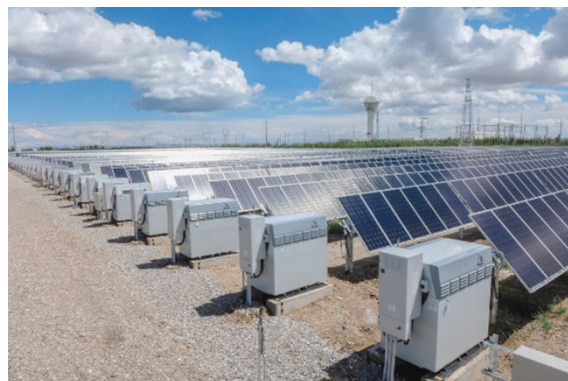
Fig. 6. a) Operational principle of the redox flow battery b) Installation for the VRB grid storage of solar energy AVALON-USA (with permission of AVALON).
