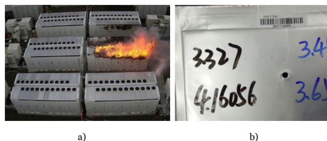
Fig. 2. a) Fire at the Victorian Big Battery LIB storage, Australia 2021. b) Faradion nail penetrated SIB pouch cell.
